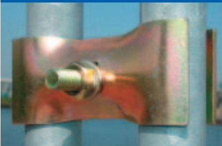
The old clamp. Functional, but easy to open using conventional tools.
